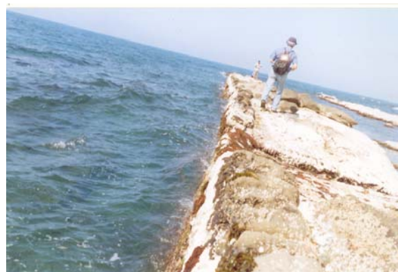
Figure 2. Rocks raised after the main shock suggesting the uplift of the coast line (Boumerdes).
